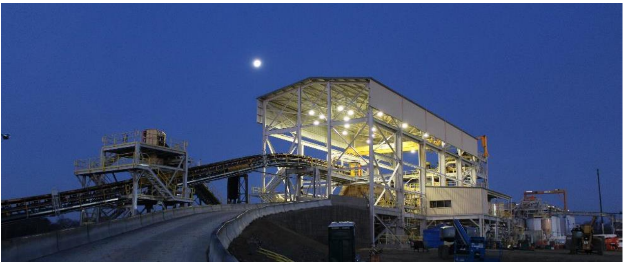
Figure 1 – Haile Gold Mine Grinding Circuit at Night
